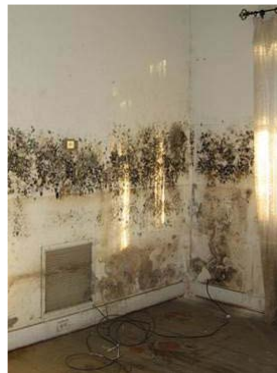
After flood waters recede, dangerous mold spores can begin to grow within 24 to 48 hours on a variety of household surfaces. Photo courtesy of Wikimedia Commons.
