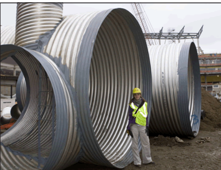
Left: Molly Gallatin of the Twins Communications Department by the 12-foot-diameter culverts. Right: The ultrafiltration system has three skids, each containing two sets of four vessels.
