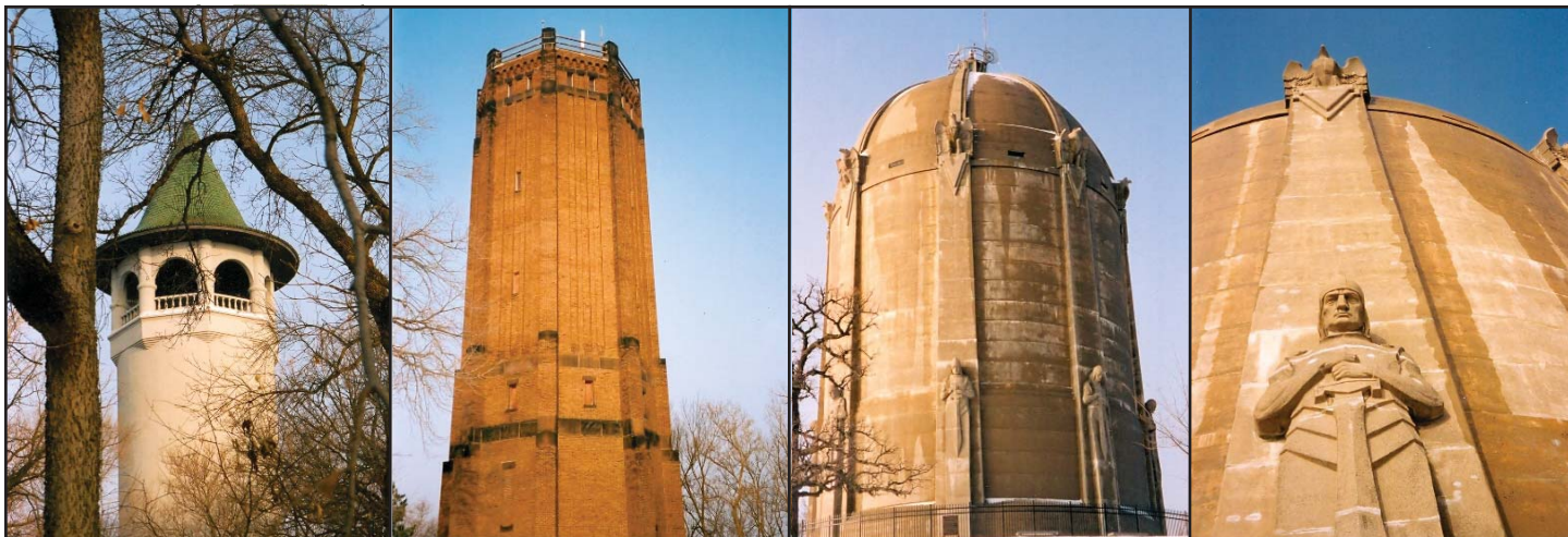
From left to right: the Prospect Park tower, the Kenwood tower, and the Washburn tower, along with a closer look at one of the “guardians of health” and the eagle at the base of the dome.
