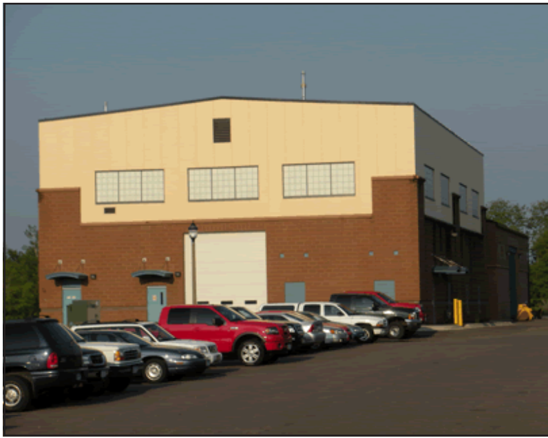
The granular activated carbon plant, on Hadley Avenue in Oakdale, treats water from Wells 5 and 9, which are to the south of the facility.
