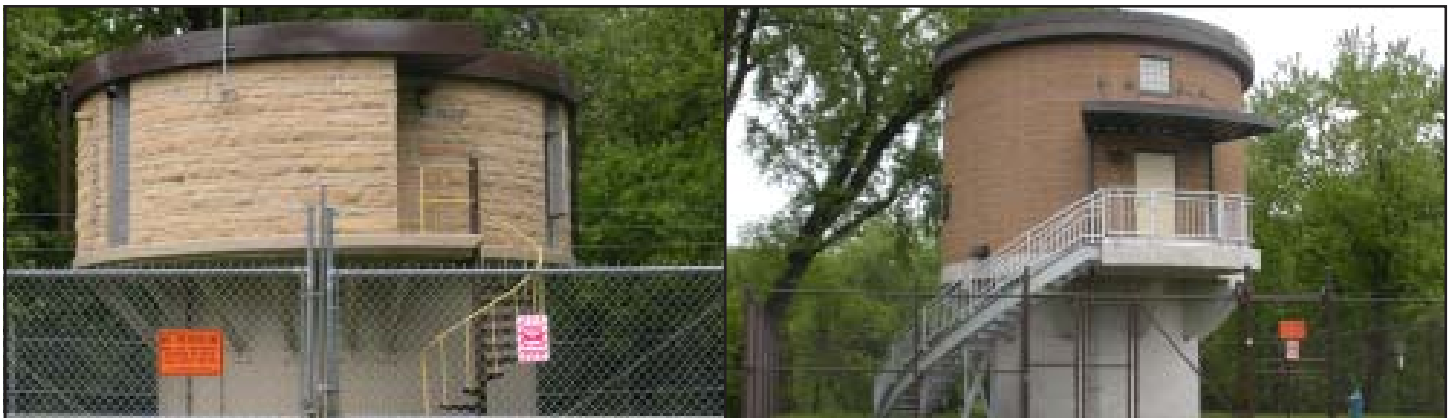
The Ranney collector wells: the existing well is on the left, new well on the right. Details on the open house that the city of Mankato will have at its new water plant in the spring of 2011 will be posted at http://www.mankato-mn.gov .
