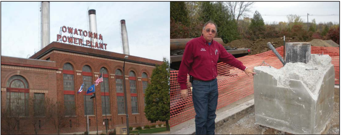
Owatonna Public Utilities was flooded in September 2010. The water utility offices moved into unflooded portions of the power plant. At right, Myron Volker points to the level the water rose to on the pump base for Well 4. The pump base had been raised earlier in 2010. It has since been removed, and the ground level raised for both Wells 4 and 2.
