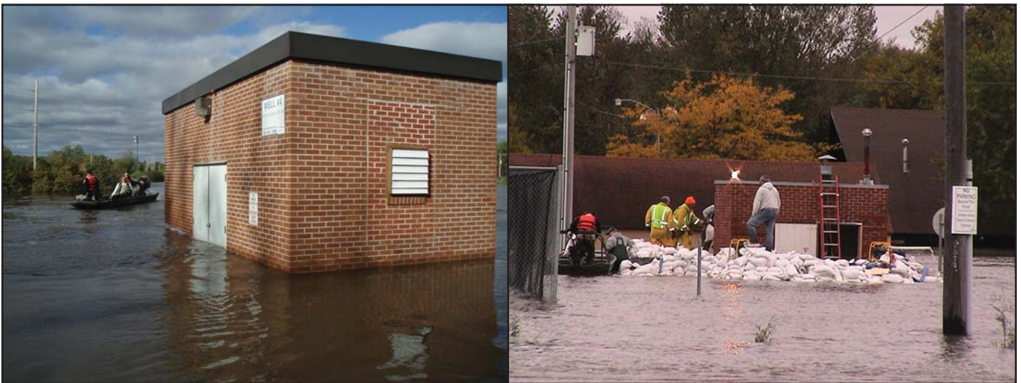
Left: Well 4 survived the 2010 flood because its pump base had been raised earlier in the year; with Well 4 out of danger, city crews and local volunteers were able to concentrate sand-bagging efforts on Well 2 (right).
