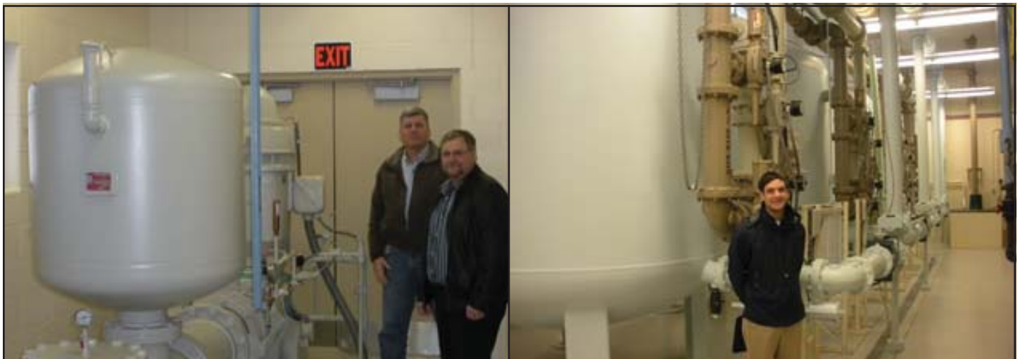
Left: Mark Peine and John Zgoda of Hastings by Well No. 5. Right: Todd Butz by the four anion-exchange filters.
