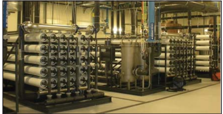
Above: Pete Moulton and Kris Swanson outside the new Broadway Avenue plant. Below: Inside the plant are three skids of reverse-osmosis vessels.
