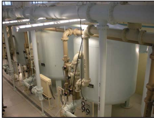
Above: An overhead look at the filters. Below: the booster pumps.
