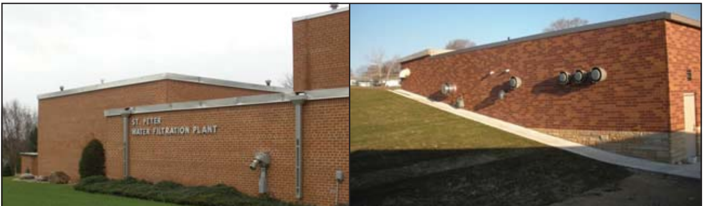
The soon-to-be demolished Jefferson Avenue plant is on the left. On the right is the new building, housing the reverse-osmosis filters, at the Saint Julien plant.
