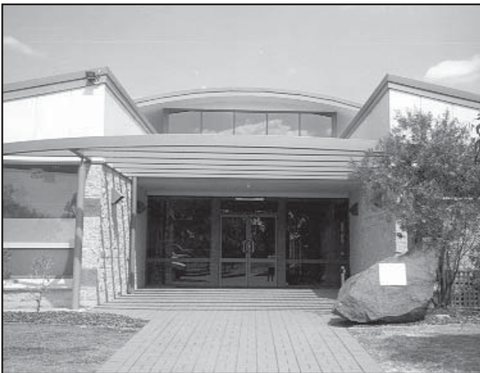
The Prospect Water Filtration Plant, which opened in 1996, is one of the largest direct filtration plants in the world.
