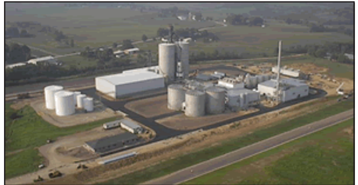
An ethanol plant. Photo courtesy of Badger State Ethanol.
