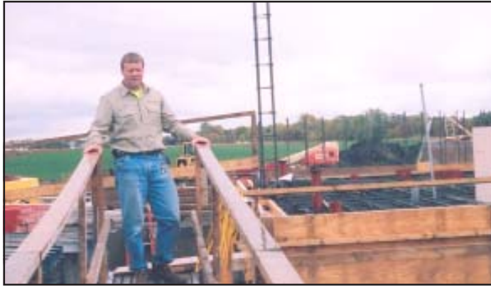
Joe Mergen at the construction site for the new water plant.
