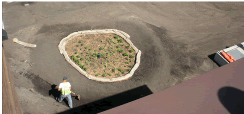
The Burnsville plant features a rain garden fed by water from the roof.
