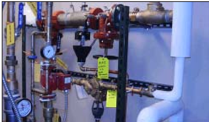
The backflow preventers for the boiler feed and cistern water (left) and the manifold for the in-floor heat tubing (right) at the Schaar’s Bluff Gathering Center in Nininger Township.
