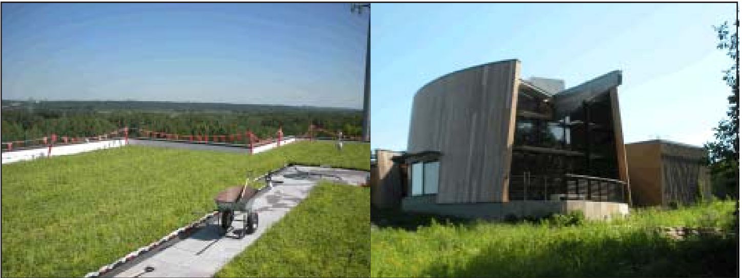
Left: The green roof on the expansion of the Burnsville Water Treatment Plant. Right: Schaar's Bluff Gathering Center
