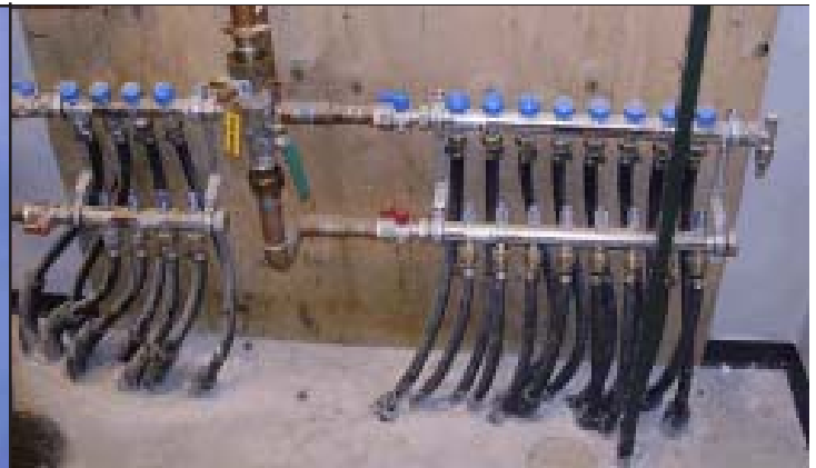
The backflow preventers for the boiler feed and cistern water (left) and the manifold for the in-floor heat tubing (right) at the Schaar’s Bluff Gathering Center in Nininger Township.
