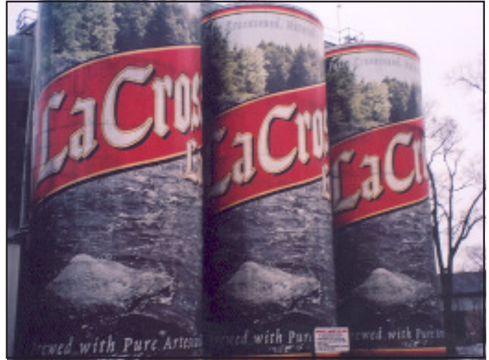
The storage tanks of City Brewing Company, which hold beer, are decorated to make them the "World's Largest Six-Pack." However, the brewing business in La Crosse, Wisconsin, has declined in recent years, enabling the city to receive wastewater from LaCrescent, Minnesota, across the river.
