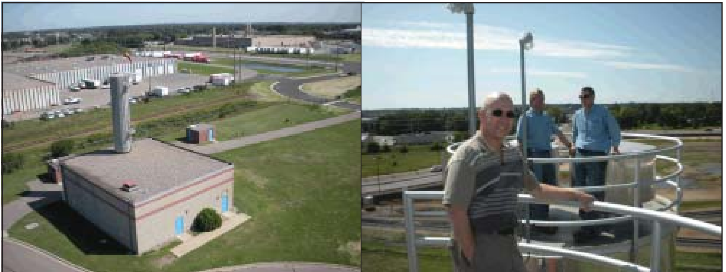
Atop the stripping towers, a look at the old plant (left). In the photo to the right, Minnesota Department of Health engineer Jon Groethe is in the foreground; Dale Warzecha and Dale Marthaler of Waite Park are in the background.
