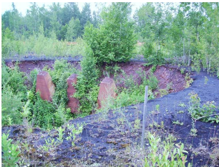
The main shaft of the abandoned Utica Mine Extension. Pictured are the concrete pillars which supported the former mine hoist. (Photo Courtesy of DNR.)
