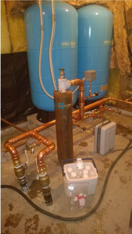
**Well and new lead-free plumbing in well house in Scandia, Minnesota. First draw water samples collected for lead analysis by MDH at 4 a.m.**
