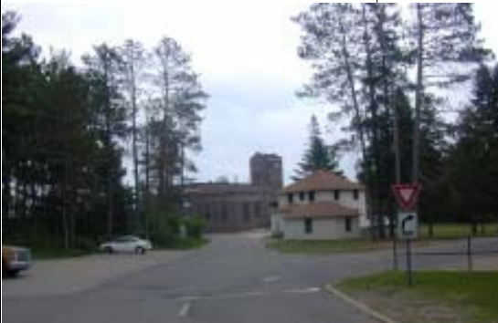
This view at the northeast side of the main building campus shows the 1925 Engineer's Cottage at right, with the 1923 Powerplant beyond.
