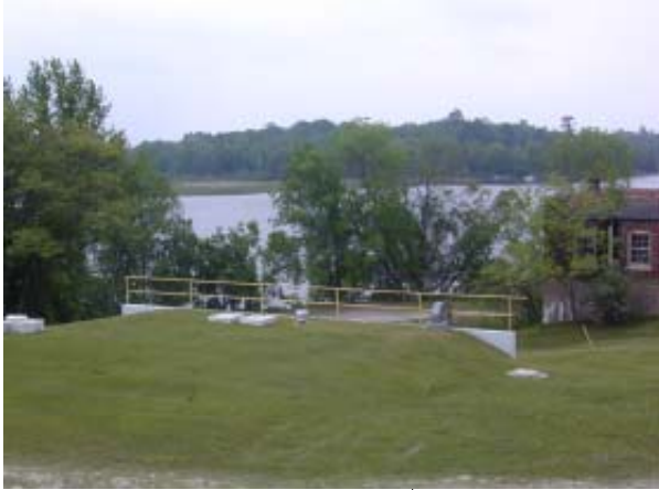
Old Pump House building near lakeshore beyond new water pumping building in foreground
