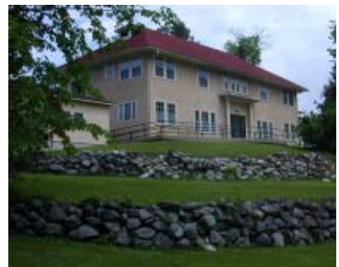
The 1915 Staff House borders on a steep hillside above Shingobee Bay, shown here adjacent to the fieldstone Retaining Wall built in 1933-34.
