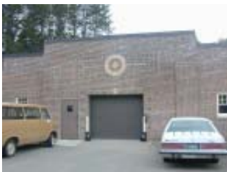
1934 Power Plant Garage
