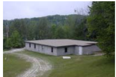
1967 Lime Storage Building
