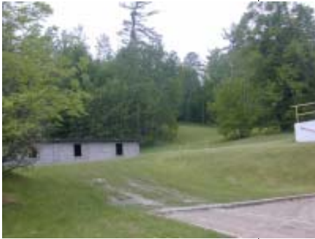
Sludge drying building near lakeshore (new water pumping building at right)
