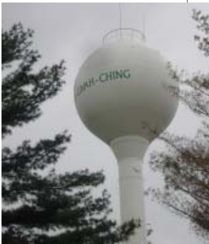
The 1986 water tower, located near Hall Memorial Pavilion, served the greater water needs of the AGCC campus of that time.
