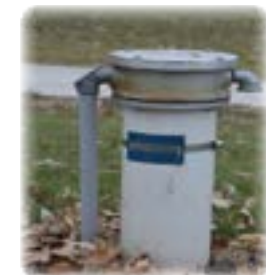
Well in good condition
