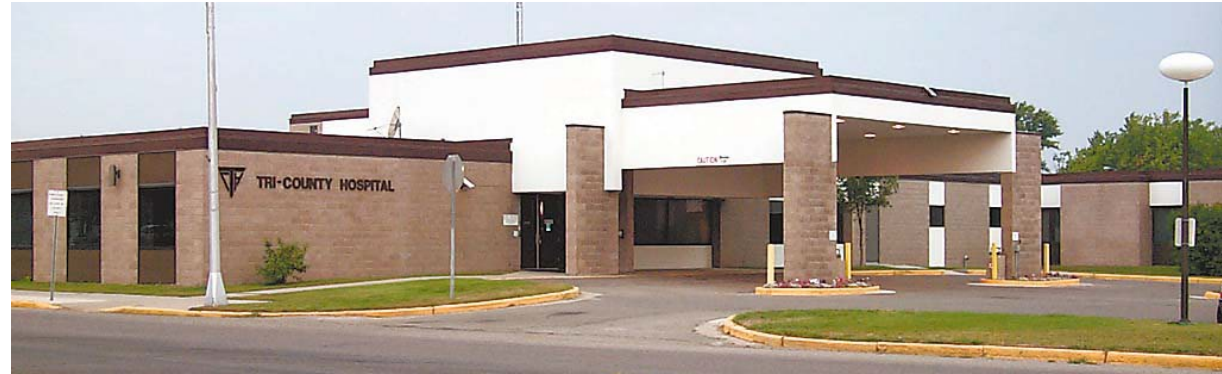
Construction begins on new hospital across the street from Wesley in 1972 and opens in 1974
