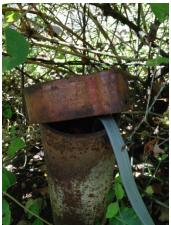
Figure 5: Coliform bacteria-positive well lacking watertight and vermin-proof cap/cover
