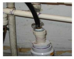
Softener discharge drain line directly plumbed to a sewer
