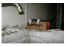
Placing the softener discharge drain line into a sink with an air gap
