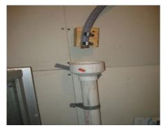
Softener discharge drain line with air gap
