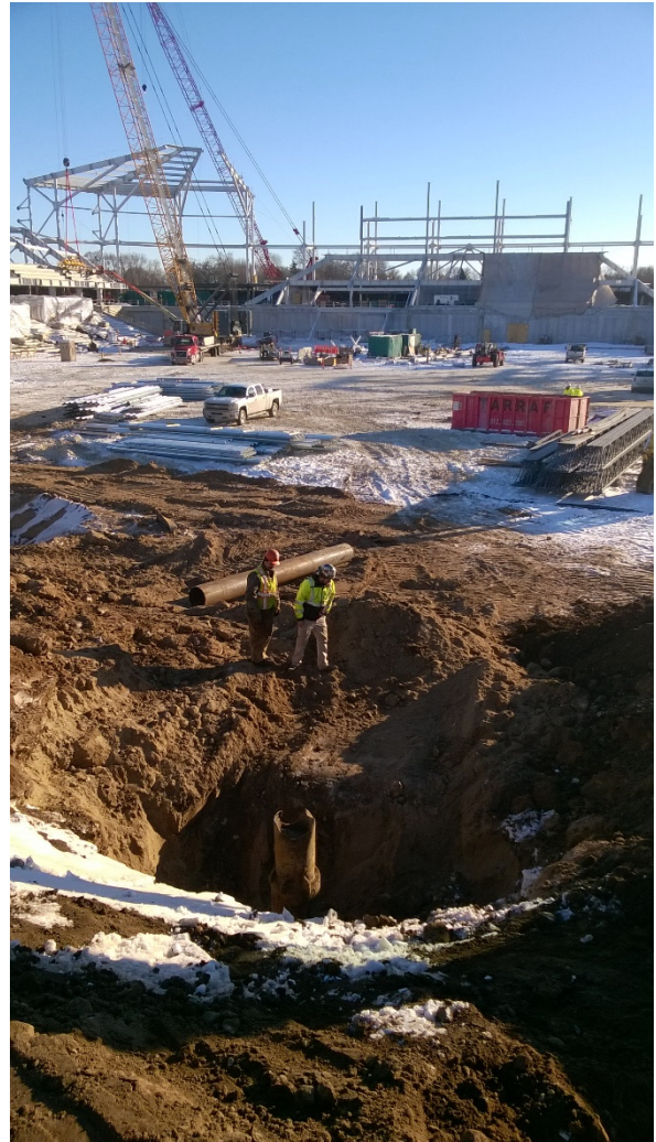
Unsealed, 20-inch by 16-inch, steel cased well located by the Minnesota Department of Health and uncovered by Mortenson Construction, at the MLS stadium site, St. Paul, Minnesota, 2018.
