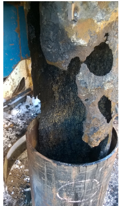
Corroded portion of 16-inch diameter liner casing being removed from within 20-inch diameter, outer well casing.
