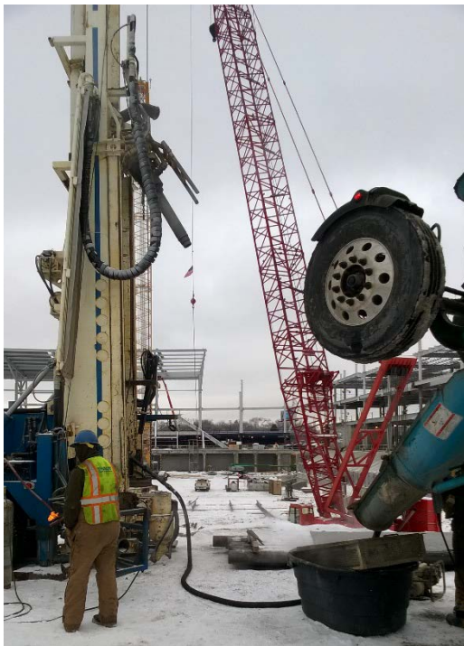
Well being permanently sealed with 45 cubic yards of "neat-cement" grout.
